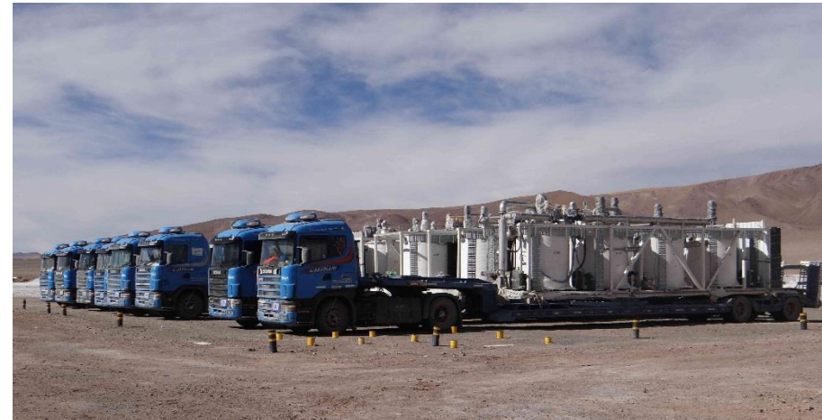
Part of the Demonstration Plant delivered to site at Rincon
