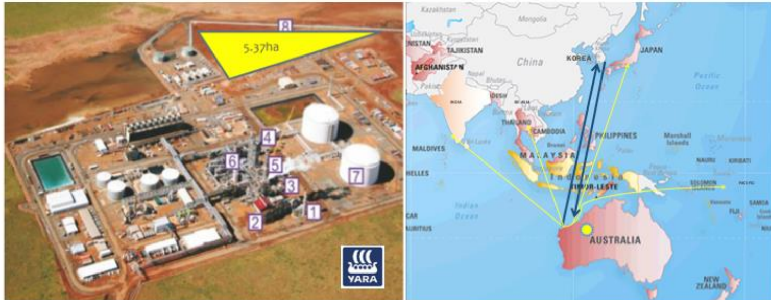
Yara Pilbara Ammonia Plant - Dampier, Western Australia
